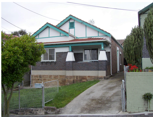
Figure 33.21 and 33.22. These two examples have both been modified by the replacement of timber windows with aluminium frames but otherwise demonstrate a substantially intact exterior. The very modest scale of these bungalows has resulted in the main door being located on the side facade to save the space otherwise occupied by a central hallway. The side access can be seen in these photographs.
