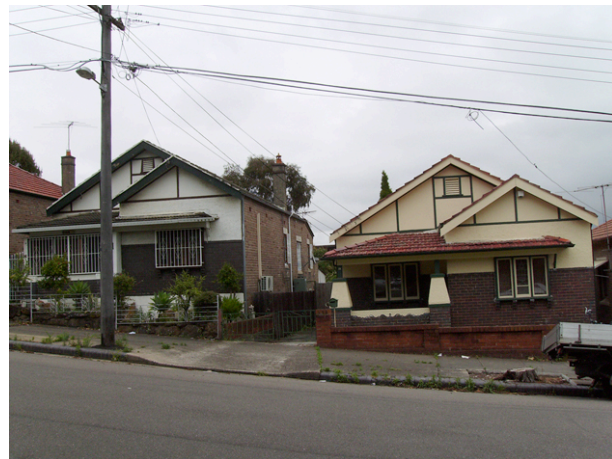
Figure 33.10. Most of the houses within the area are a simplified version of the usual Californian bungalow, with a hipped roof over the porch and front window instead of the more common triple gable form. Their access is provided through a door on the side façade – both a space-saving device for these small cottages as no central hallway was required; and reflecting the emerging importance of the motor car as the primary method of arrival. Each is offset on its lot to allow a side driveway.
