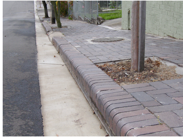
Figure 33.8. An important element of the Wells Avenue streetscape is the survival of the 1930s Depression Employment Relief Scheme brick paving with bull nosed edging. Although patched in places its herringbone patterning adds an important texture to the streetscape.
