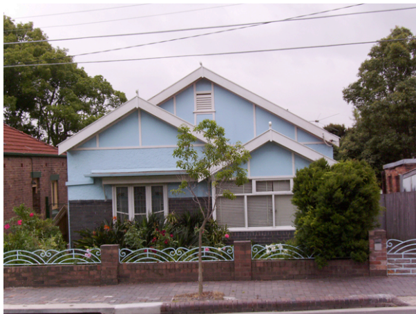
Figure 33.27. This house has been modified through the enclosure of the verandah and the painting of the plasterwork in a bright colour. The underlying form is intact however and the changes are potentially reversible.
